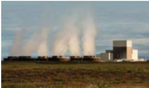
Columbia Generating Station (1,207 MW)
