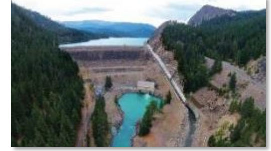
Tieton Hydroelectric Project (15 MW)
