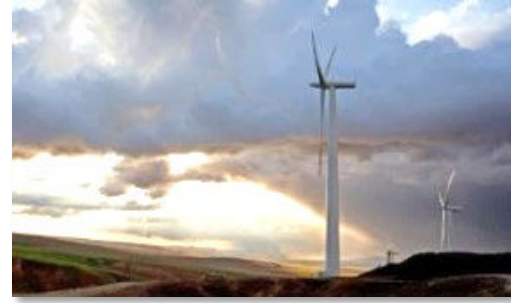
Nine Canyon Wind Project (96 MW)
