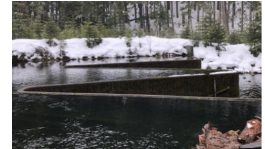
Stone Creek Hydro Project (12 MW)
